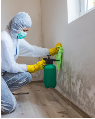
(household mold damage)
